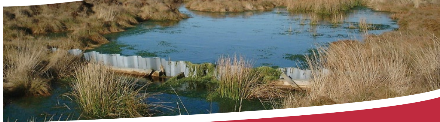
Damming drains to help regenerate the bog
