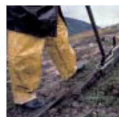
Footpath repair, Coire Etchachan, Cairngorms
